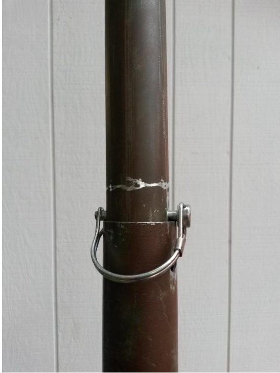
Extended section held in position by pin
